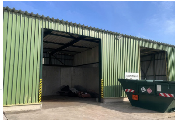
Fig.: Washing box for cleaning elements ("pigs") at PS 1 Budkovce.
