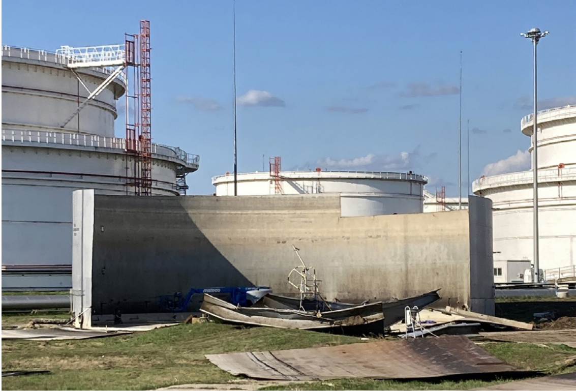
Fig.: Removal of old fire water tank.
