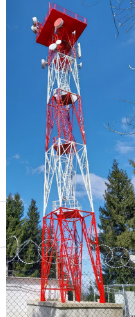
Fig.: As part of the reconstruction of inspection chamber facilities along the pipeline route, the roofing with accessories and the facades of selected inspection chambers were restored. Within the reconstruction of RR Point masts, selected masts were reinforced, and the coating was renewed, which also as daytime aviation obstruction marking – the photograph shows RR point mast at Detvianska Huta location.
