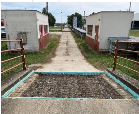
Fig.: Photographs from the reconstruction of the bridge approach sections at PS 1 Budkovce.
