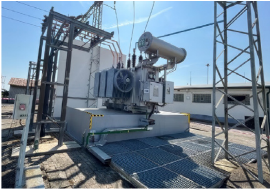
Fig.: Containment pits of T101 and T102 transformers at PS 1 Budkovce after reconstruction.
