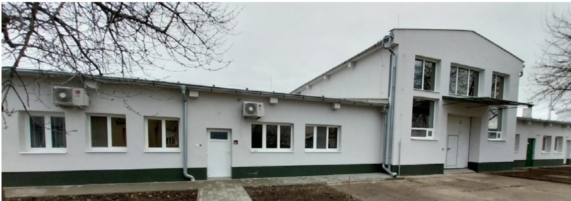
Fig.: As part of reconstruction of Facility 080 - 100 MTZ warehouse at PS 4 Tupá, a roof, facade, and windows were renovated.
