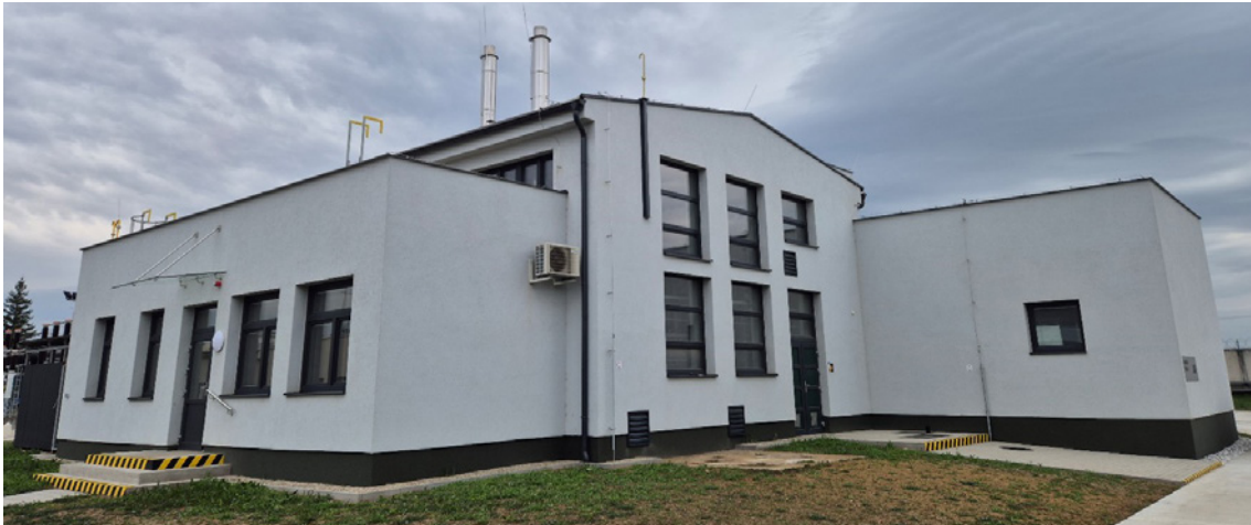
Fig.: Renovated premises at PS 4 Tupá for staff of Department of Long-distance Pipelines and Cathodic Protection.
