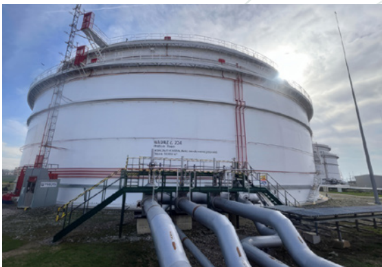
Fig.: Oil tank No. N234 at PS 1 Budkovce after coating renovation.
