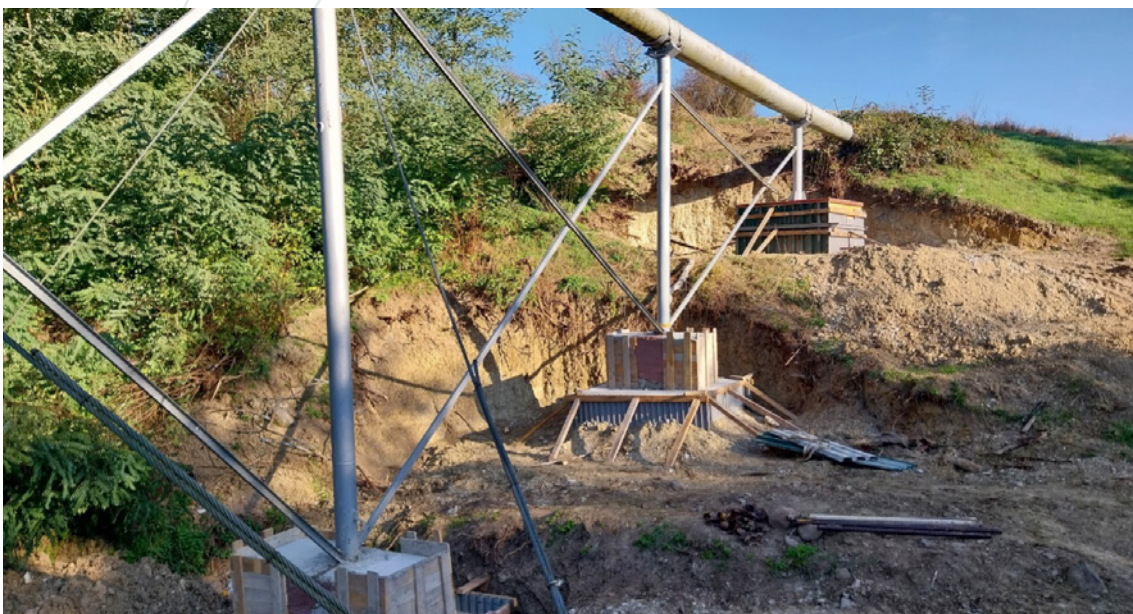
Fig.: Photograph from the reconstruction of aboveground section of Ďurkovce along the oil pipeline route.
