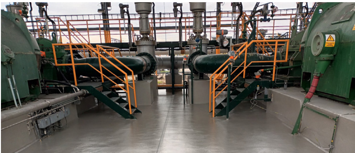
Fig.: Within IA No. 52401 – Reconstruction of loading area in ČS 221 and repair of support bases at PS 5 Bučany, the floor in oil pumping station No. 221 at PS 5 Bučany was also renovated.
