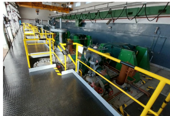
Fig.: Reconstructed floor in oil pumping station No. 221 v PS 4 Tupá.
